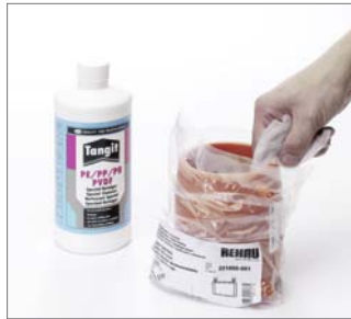
Fig. 114 Only remove the FUSAPEX electrofusion fitting from its bag immediately prior to welding. Clean the fitting as required.
