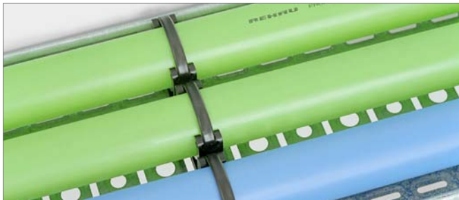
Fig. 130 RAUPEX pipes installed in a cable carrier system
