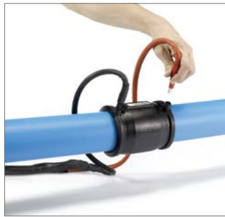
Fig. 51 13. An acoustic signal sounds once the welding process has been completed. The display reads "OK".
