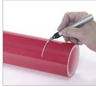
Fig. 111 For marking, employ a pen with a different color to that of the pipe.
