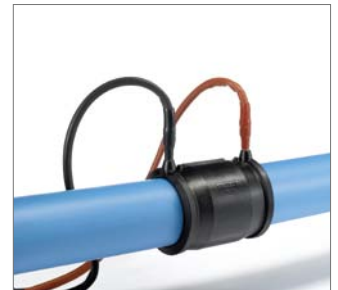
Fig. 49 11. Check the alignment and insertion depth. There must be no strain exerted during welding. If necessary, employ round-backed clamps or pipe clamps.
