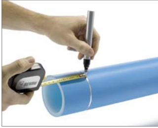
Fig. 65 Use a PE pen in a contrasting color for marking.
