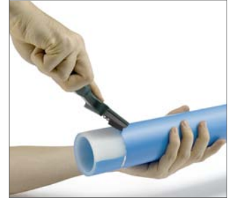
Fig. 41 3. Using the manual scraper, completely remove the coating. Do not go beyond the marking. The chip thickness should be approx. 0.2 mm.
