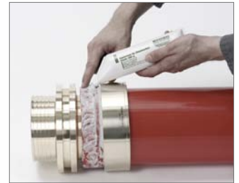
Fig. 32 7. Apply REHAU lubricant uniformly around the entire pipe circumference in the connection area.
